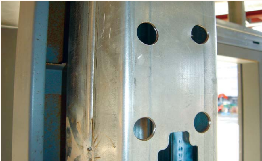
Access holes are drilled in the welded box sections to attach the HMF into the metal-stud framed opening.
