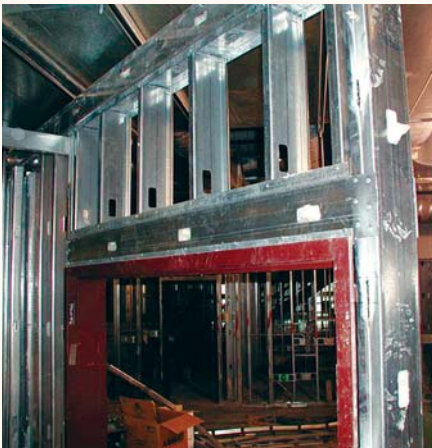
Studs and tracks are commonly hand-cut to size, dog-eared on each end, fastened with multiple screws and often welded, depending on the skill and preference of the installer.
