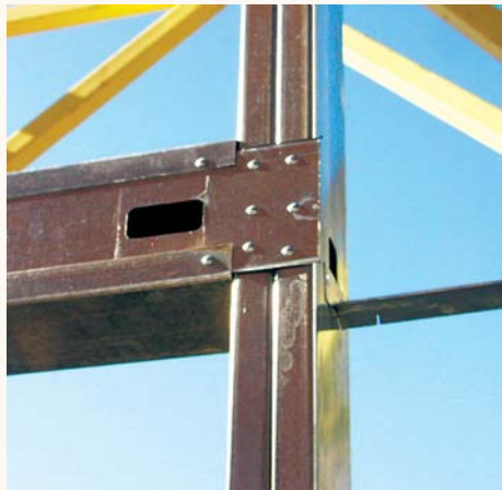
Studs and tracks are commonly hand-cut to size, dog-eared on each end, fastened with multiple screws and often welded, depending on the skill and preference of the installer.
