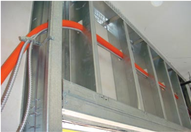
These two photos show the interior and exterior of the opening for a sliding glass door to a terrace. The header used establishes a smooth surface for the drywall and plaster crews. There are 16 of these units on each floor of the building.
