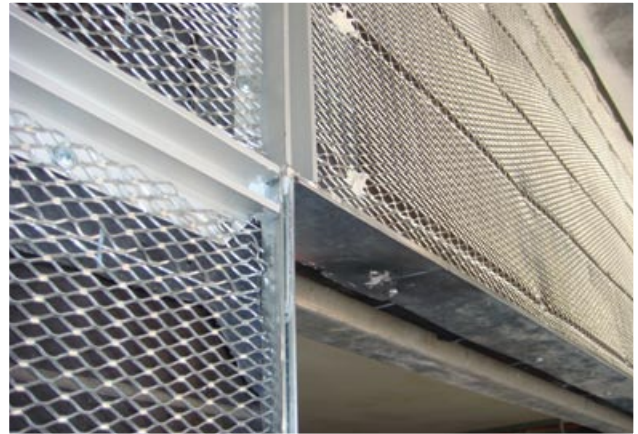
These two photos show the interior and exterior of the opening for a sliding glass door to a terrace. The header used establishes a smooth surface for the drywall and plaster crews. There are 16 of these units on each floor of the building.
