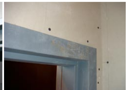
Because the ProX header allows drywall to lie flat against the steel framing, significant time is saved in the taping and finishing phase. Shown at left is steel framing without drywall; in center, drywall installed flat against the steel; and at right, clean and flat drywall around the door frame and in the corner.
