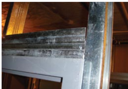
Because the ProX header allows drywall to lie flat against the steel framing, significant time is saved in the taping and finishing phase. Shown at left is steel framing without drywall; in center, drywall installed flat against the steel; and at right, clean and flat drywall around the door frame and in the corner.
