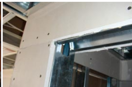
Because the ProX header allows drywall to lie flat against the steel framing, significant time is saved in the taping and finishing phase. Shown at left is steel framing without drywall; in center, drywall installed flat against the steel; and at right, clean and flat drywall around the door frame and in the corner.
